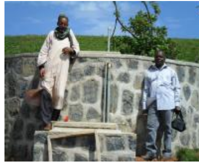
Edwin Visi, our consultant engineer and a villager near a finished storage tank.
